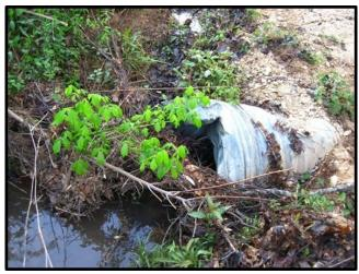
Figure 23.—Example of poor inlet/outlet condition (blocked).
