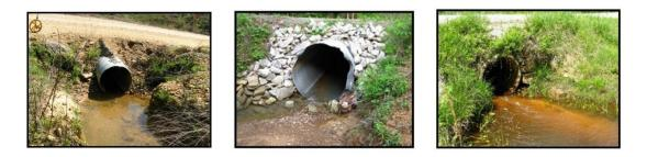
Figure 25.—Comparison of poor, fair, and good outlet conditions
