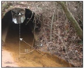
Figure 21.—Example of upstream skew angle >30° (Witmer, 2009).
