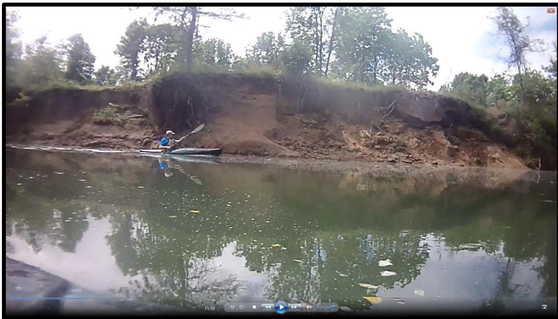
Figure 7: Level 5, Very Poor Condition: Banks with the highest erosion potential and steep bank angles. Evidence of active bank failure, with very little stabilization from vegetation. Obvious impacts from cattle, agriculture, and industry with no connectivity to flood plain. Contribution of sediment is very high in these areas.
