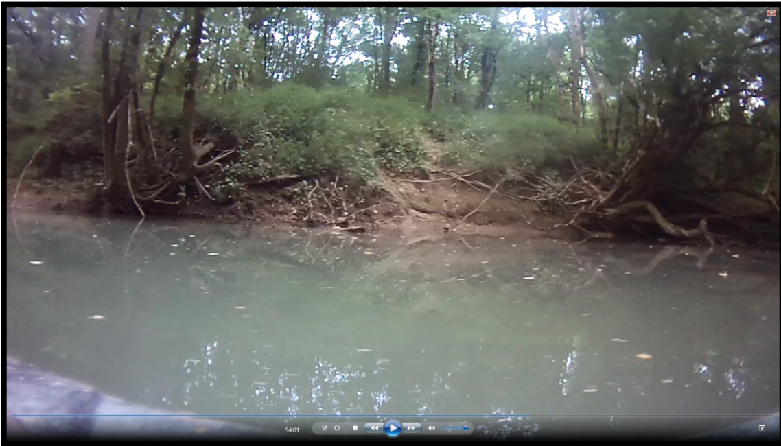
Figure 7: Level 3, Fair Condition: Banks showing moderate erosion impact with limited access to flood plain and variable surface protection. Potential impacts affecting water quality and aquatic habitat. Immediate action is not necessary.
