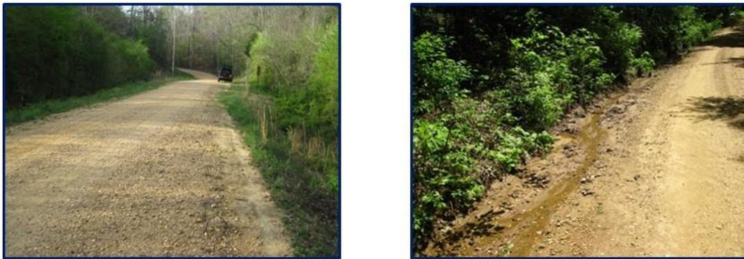
Figure 26.—Comparison of a well vegetated ditch in good condition and a bare soil ditch on a steep slope in poor condition.
