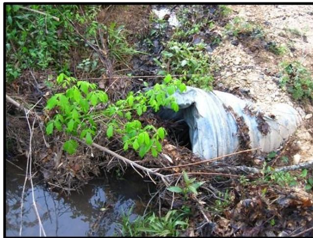
Figure 23.—Example of poor inlet/outlet condition (blocked).
