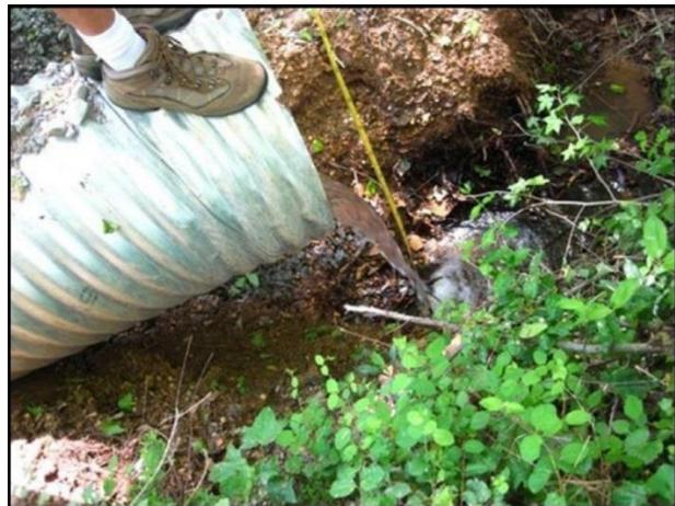
Figure 22.—Example of poor crossing structure fill condition.
