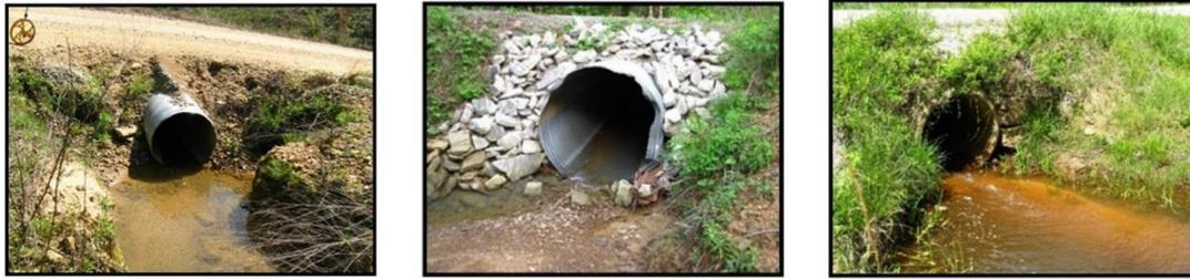
Figure 25.—Comparison of poor, fair, and good outlet conditions
