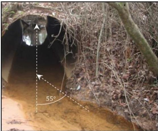
Figure 21.—Example of upstream skew angle  $>30^\circ$  (Witmer, 2009).
